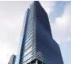
Fujitsu General Electronics (Suzhou) Co., Ltd.
