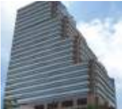
Fujitsu General (Thailand) Co.,Ltd. Bangkok Office (Thailand)
