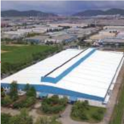
Fujitsu General (Thailand) Co., Ltd. (Thailand) Factory-2
